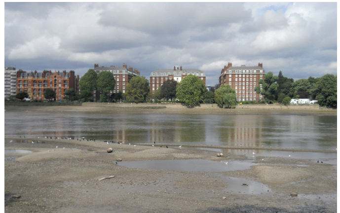
Figure 4.5: Hurlingham Court and Rivermead Court blocks lining the river's edge
