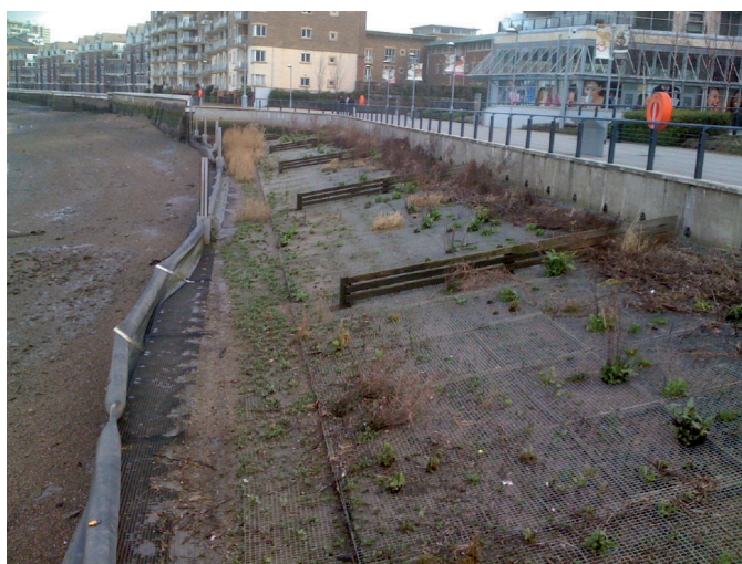
Figure 13.8: Managed retreat of the riverbank at Battersea Reach
